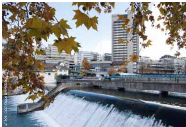
Producing green electricity from lake water in the middle of the city: the Letten power plant.
