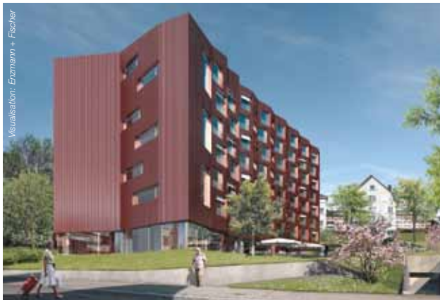
Compact building envelope, sun-facing windows, wood pellet heating: the Trotte Retirement Home
