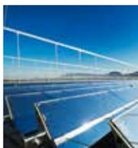
Located in the sunny Spanish region of Murcia, the Puerto Errado 2 thermal solar power plant went into operation in 2012 and is based on Fresnel technology with direct evaporation. It was constructed under Swiss management. Along with two conventional power plant blocks, the facility encompasses a solar field with around 302 000 m<sup>2</sup> of reflective surfaces.
